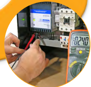
Inspection of Electrical Components
